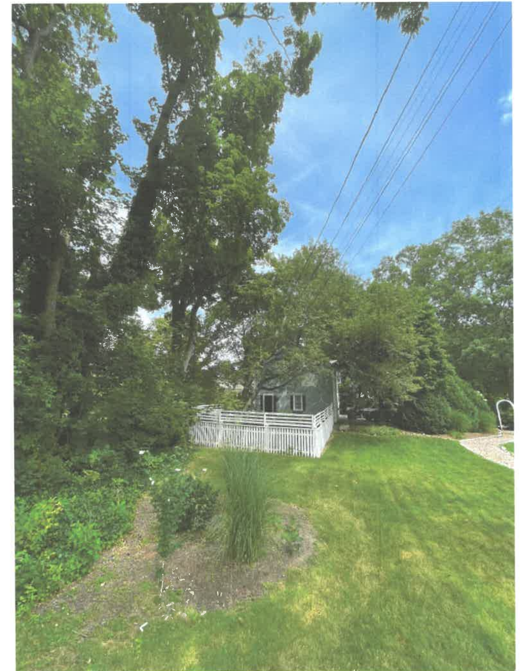
Existing Condition: From one pole located on the street three homes are currently connected. The Gagne's and the O'Donnell's power lines cross 30 Rector Street in order to connect to the existing pole at the corner of Pat's home that is located on the O'Donnell's property.
